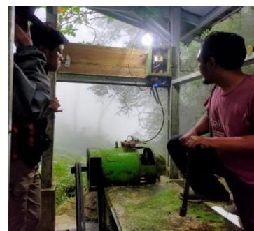
Figure 4. Installation process of IoT devices on MHP in Argamukti Village
