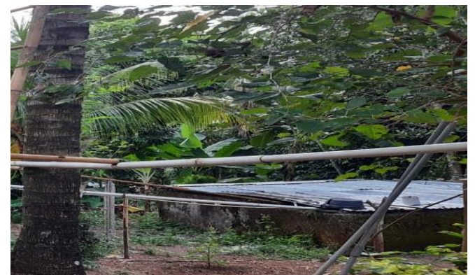
Figure 9. Rainwater Catchment Network towards the Reservoir Tank
