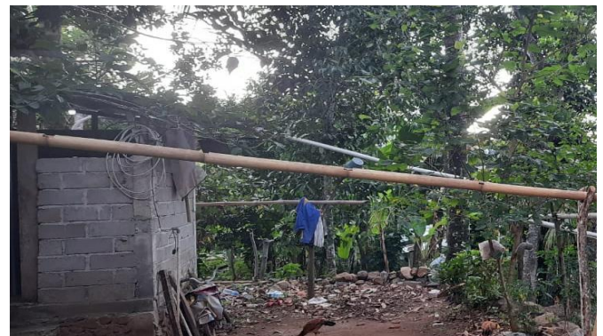
Figure 8. Water Catchment Network with Bamboo Material
