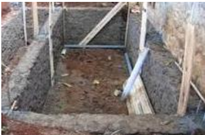
Figure 5. Rainwater reservoir made from river stone masonry
