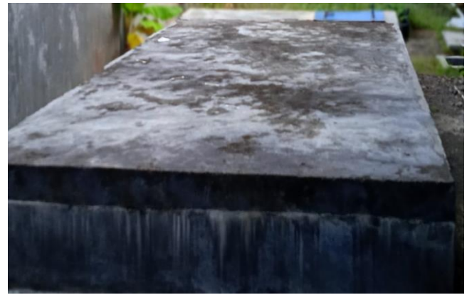
Figure 7. Reinforced concrete water reservoir
