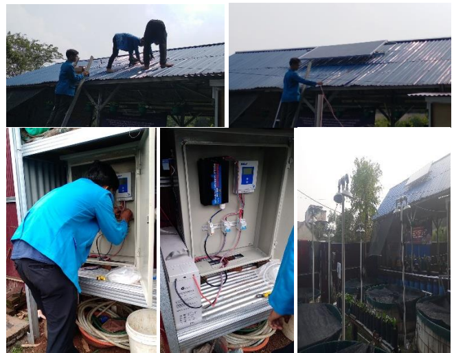
Figure 3. Results of installing solar panels, MPPT panels and light towers
