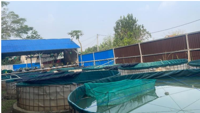
Figure 2. Conditions Before the PLTS System was Installed
