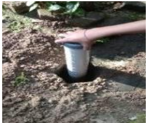
b. Inserting a pipe into the hole
