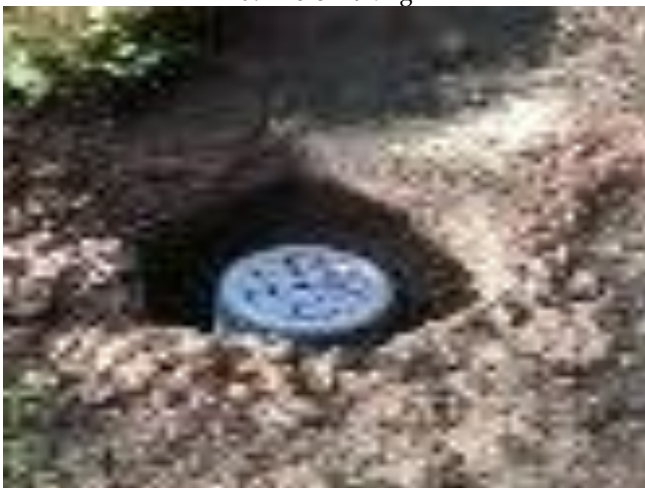
c. The pipe is installed
