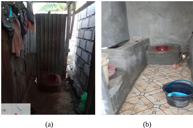
Figure 3. Toilet Documentation: (a) before repair; (b) after repair
