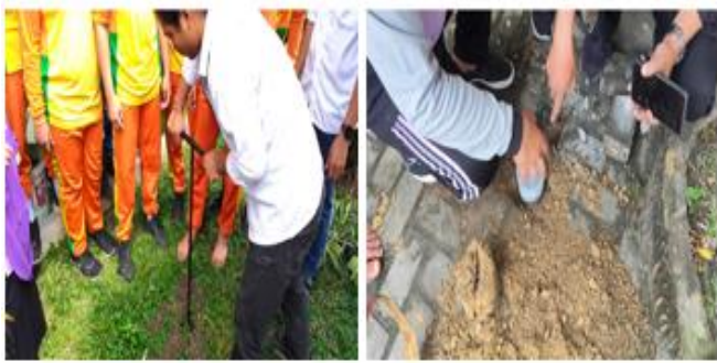
Figure 3. Biopore Hole Construction Practice
