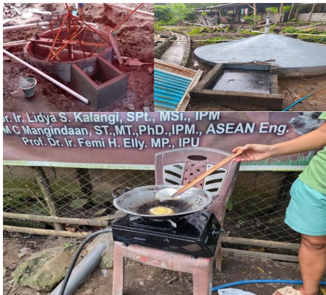
Figure 3. Stages of Biogas Digester Construction: Before, During, and After
