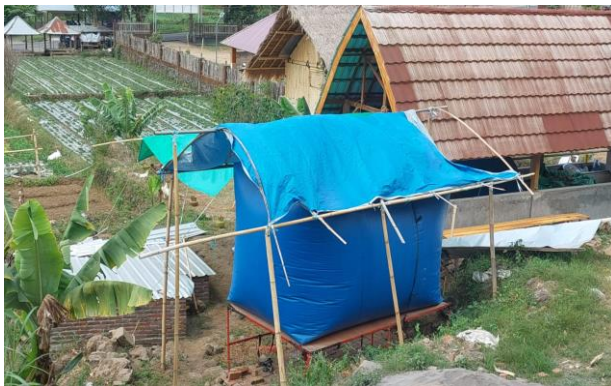
Figure 4. Biogas storage with a capacity of 12 m 3
