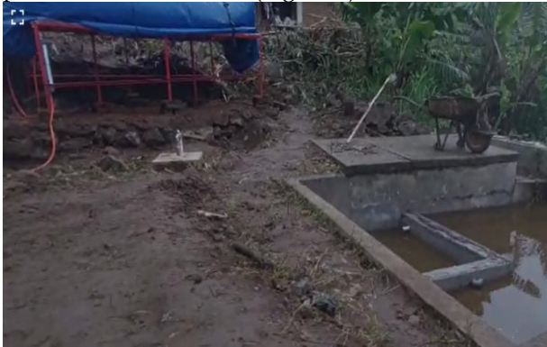
Figure 3. The biogas digester with a capacity of 8 m 3 .
